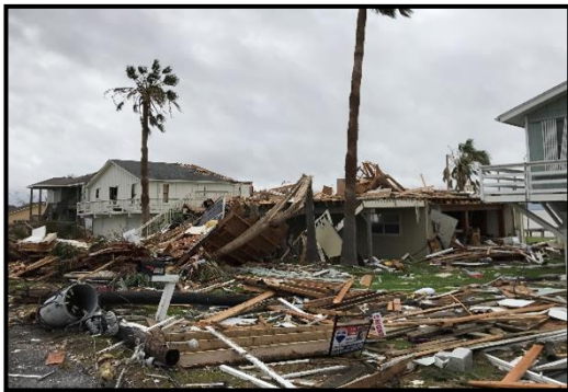
Above: Damage to the community of Copano Village in Aransas County, TX in the wake of Hurricane Harvey in 2017.
