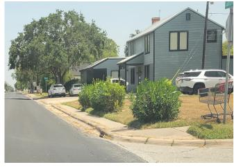
Sidewalk at curb-face with insufficient buffer from traffic on Santa Fe Street,
