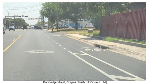
» Buffer between car traffic and bike traffic via two painted white lines, with or without diagonal cross hatching
