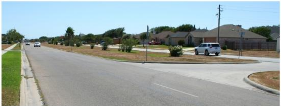
The city will remove the median on Memorial Parkway between Buddy Ganem Drive and Oak Brook Drive.
