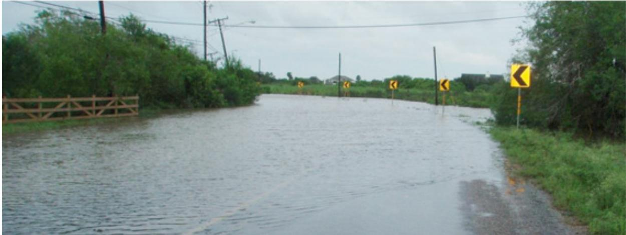
The area just south of the Oso Creek has a low spot and the design will incorporate improved drainage and raise the road to reduce flooding of the roadway. Drainage from farm land west of the Oso will also be a factor in the final engineering. Working with local property owners TxDOT will provide an optimum design for site drainage.
